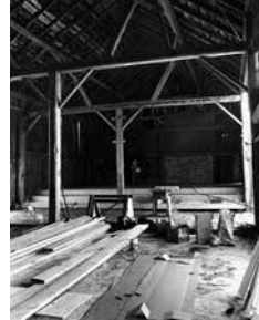
Dutton Concert Barn stage under construction, 1977.
